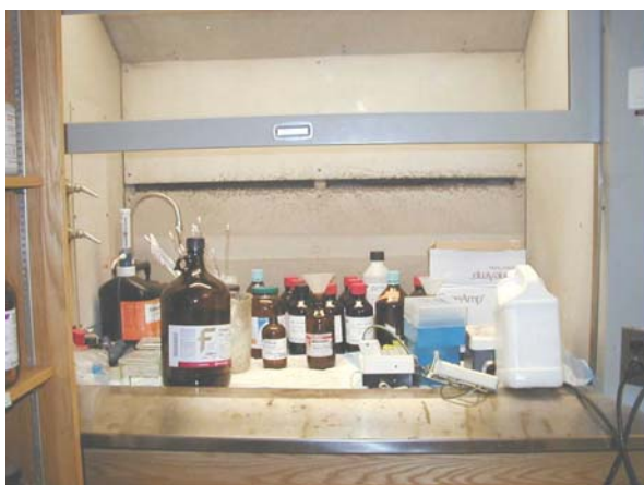
Figure 2: Improper chemical storage in a hood blocks the slot and air foil.
